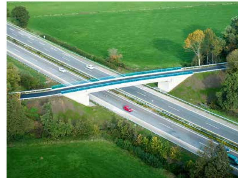
Echterhoff express bridge crossing the A3 near Hamminkeln
