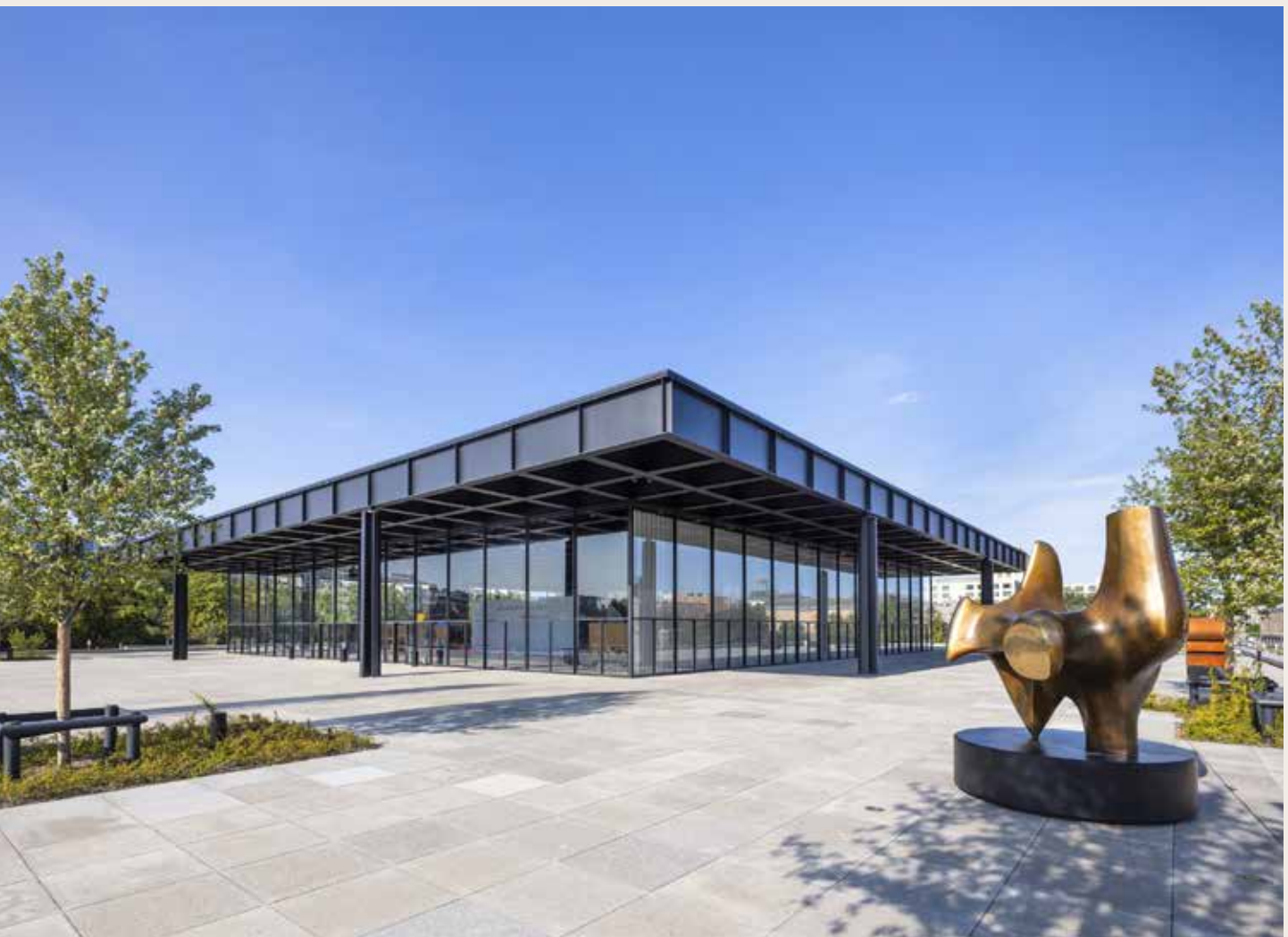
The New National Gallery of the architect Ludwig Mies van der Rohe on Potsdamer Strasse in Berlin shines again
